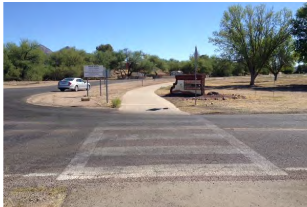
Existing Pedestrian Crossing at Pendleton Drive and Avenida Coatimundi
