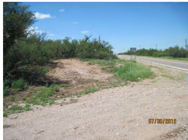
Construction of West Frontage Road Shared Use Path
