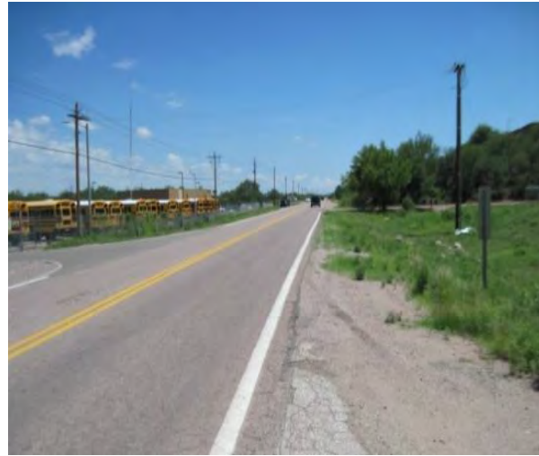
West Frontage Road looking south near Camino Lito Galindo
