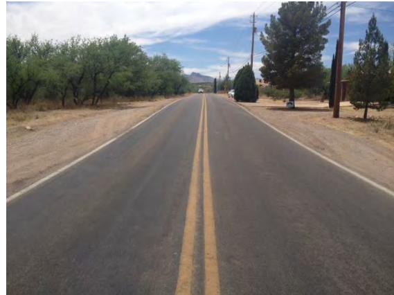
Camino Ramanote looking west
