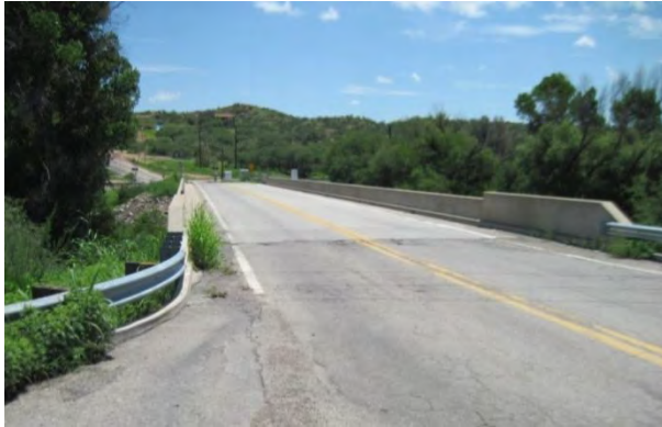
Potrero Creek Bridge on Ruby Road
